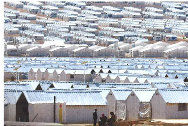
Prefabricated metal homes at the Azraq camp for Syrian refugees in northern Jordan. Photograph by Khalil Mazraawi/AFP, January 30, 2016. © Getty images.
