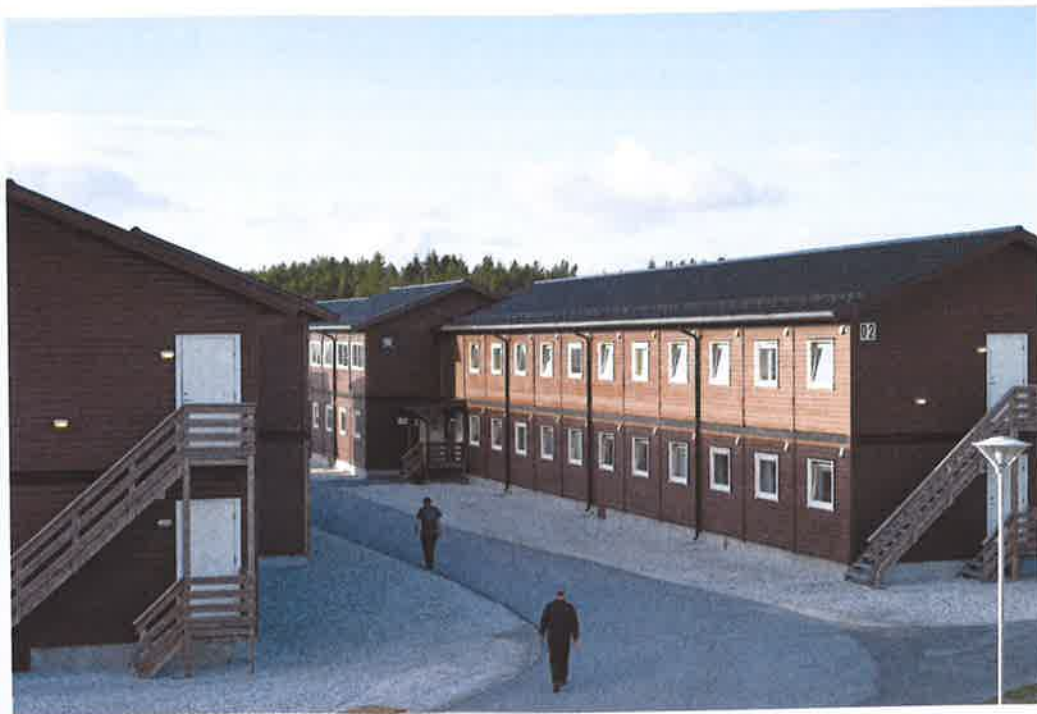
Temporary living premises for workers at Statoil Mongstad. Photograph by Helge Skodvin, 2016. Courtesy of the author.
